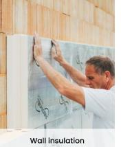
2023, a range of thermal insulation boards for cavity wall and flat roof insulation, containing 25% bio-circular raw materials and reducing  $CO_2$  emissions by an average of 43% compared to standard boards.
