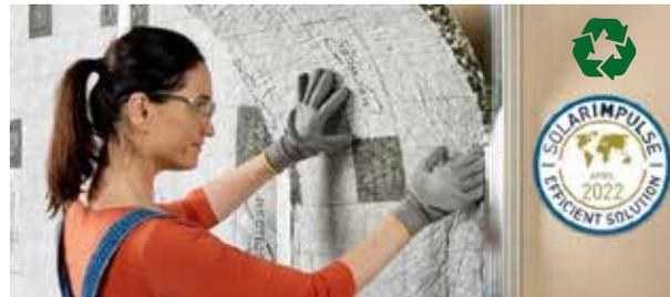
Our inner wall solutions are also made from recycled materials and are simply attached to the interior wall with a special adhesive, reducing noise by around 87%.
