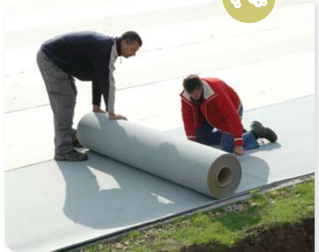
Construction of an artificial outdoor football field (Re-bounce®)
